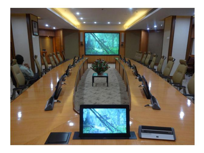
Beyerdynamic MCS-D Series digital array microphones with the beam forming Revoluto Technology is used for push to talk application with chairman and delegate microphones. The microphone button, clear button are being used based on the speaker where as priority button is associated with chairman microphone gives the full control to Chairman to either allow or mute the user.
